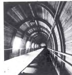
Figure 15: Formwork waling effect, conveyor interior, from Architectural Forum , March 1944.
