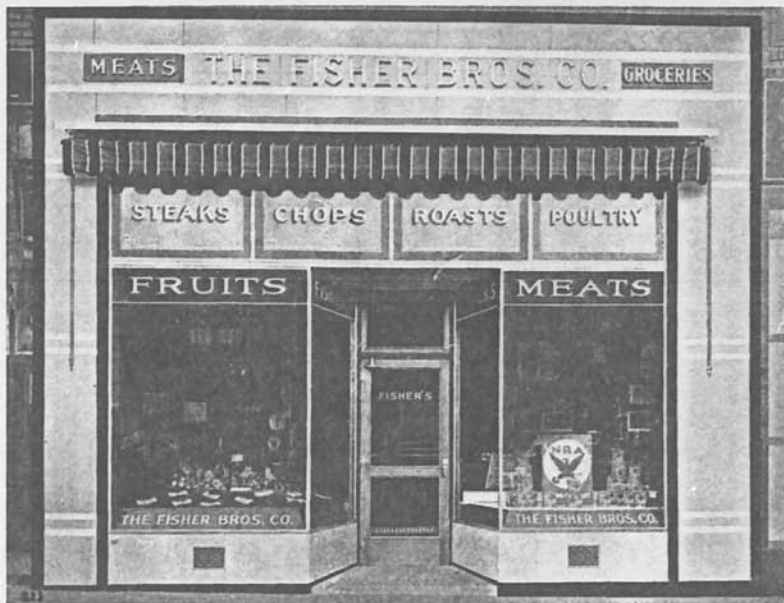
HERE IS A typical Chain Store Front in Cleveland, Ohio, constructed with Pittco Store Front Products. Notice how clean, fresh and inviting it looks, catching the eye of potential customers and welcoming them in the modern manner. Jule, White and Black Carrara Structural Glass have transformed an outmoded space into a money-making chain store site.
